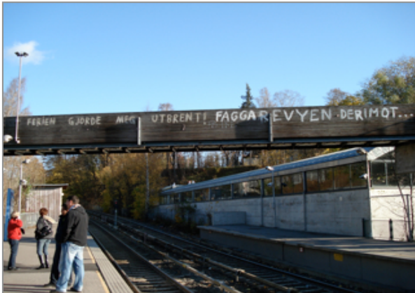
Photo 2. Pedestrian bridge over the tracks
