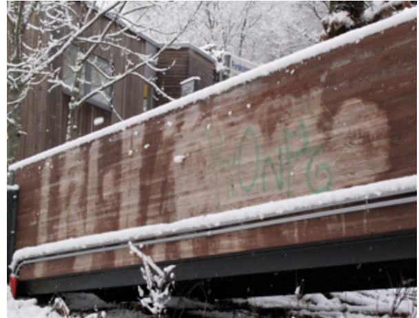
Photo 14: Traces on wooden siding
