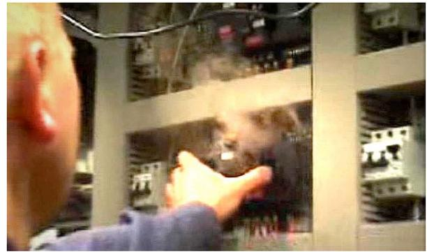
Figure 3 Preben pulling out a smoking controller out the control cabinet
