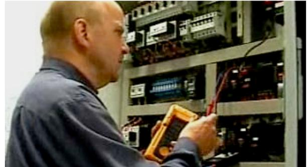
Figure 4 Preben using a volt meter to measure electric current in the control cabinet
